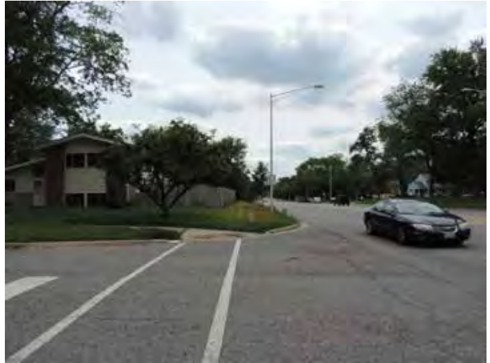
Discontinuous sidewalk on Western Avenue. Photo by CMAP staff.
