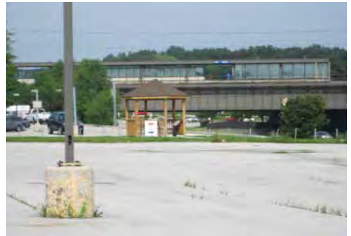
211th Street Metra Station. Photo by CMAP staff.
